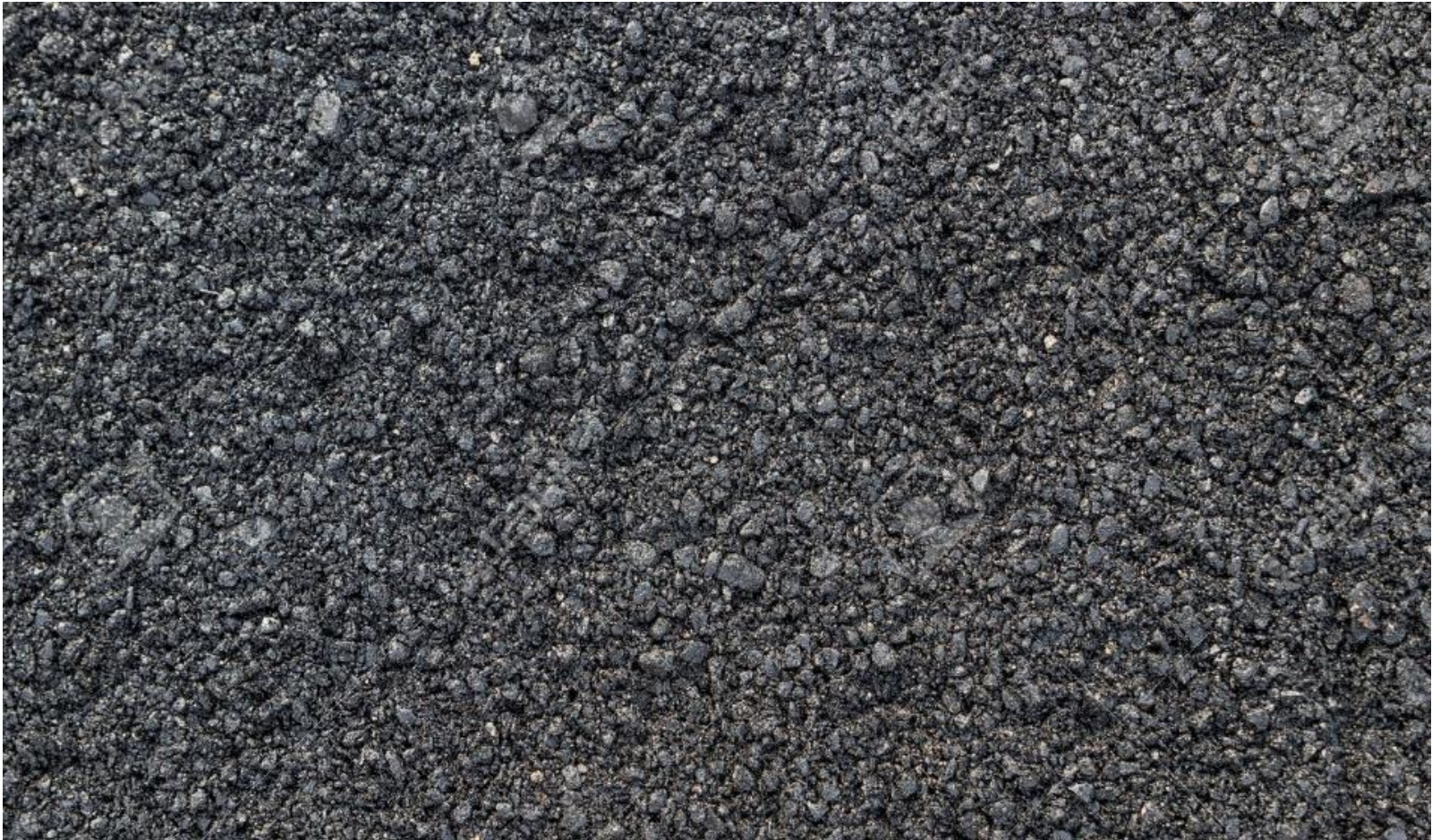
hot mix-asphalt road surface
