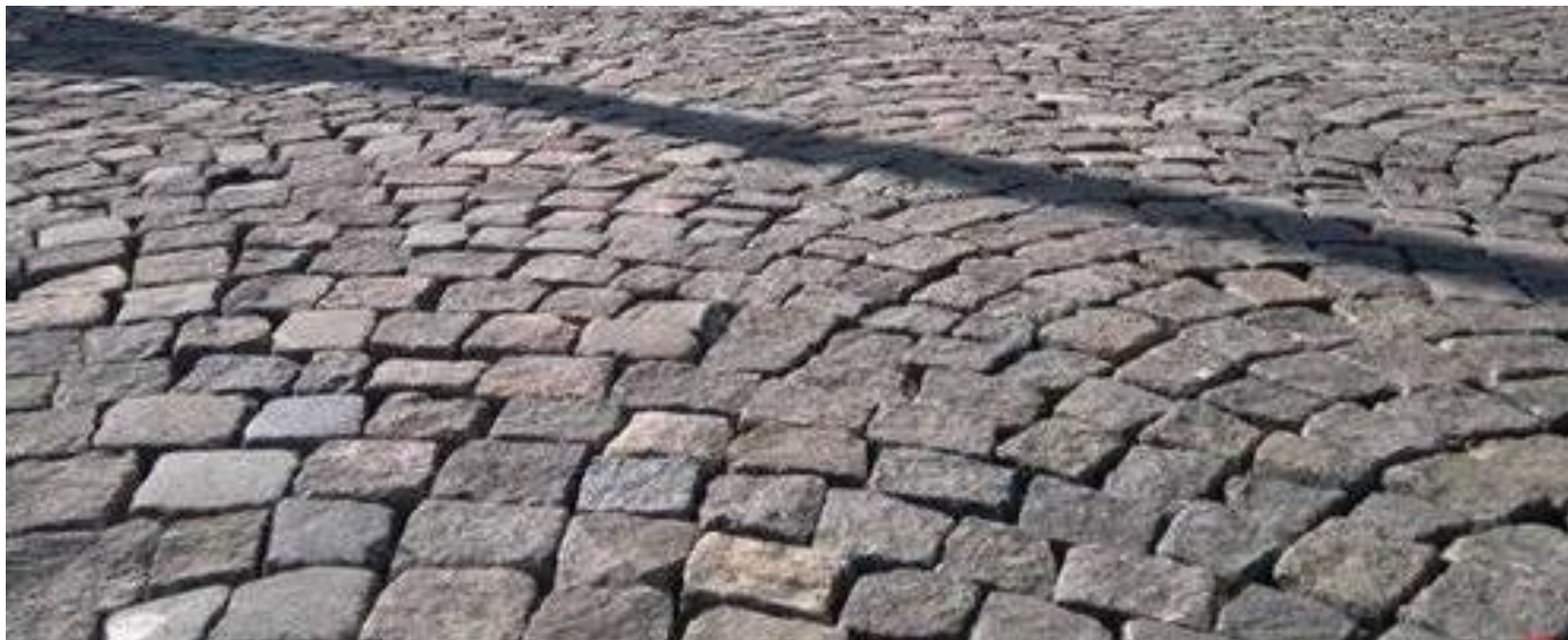
cobbles road surface
