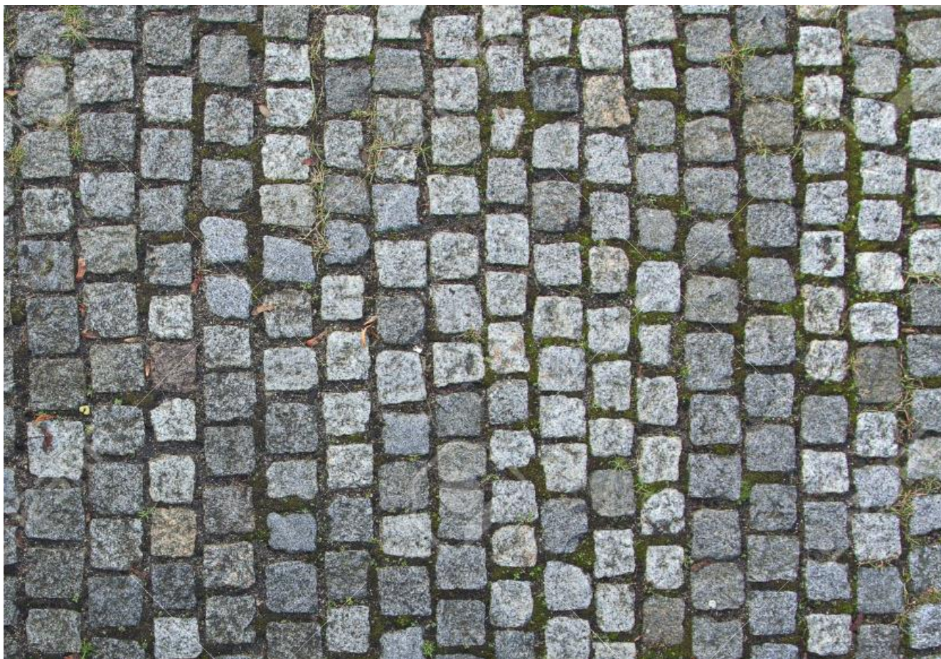
setts road surface
