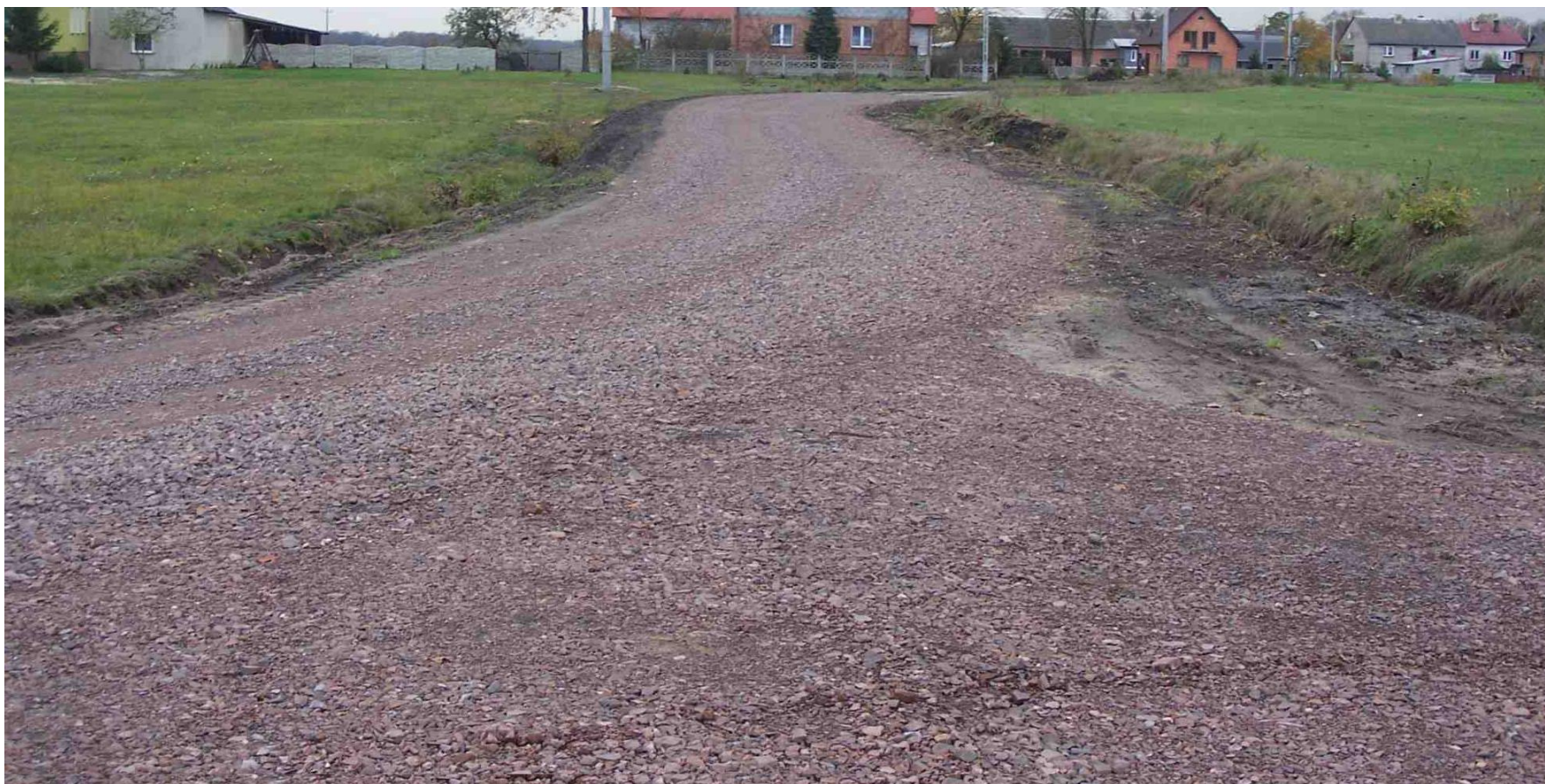
crushed stone road surface
