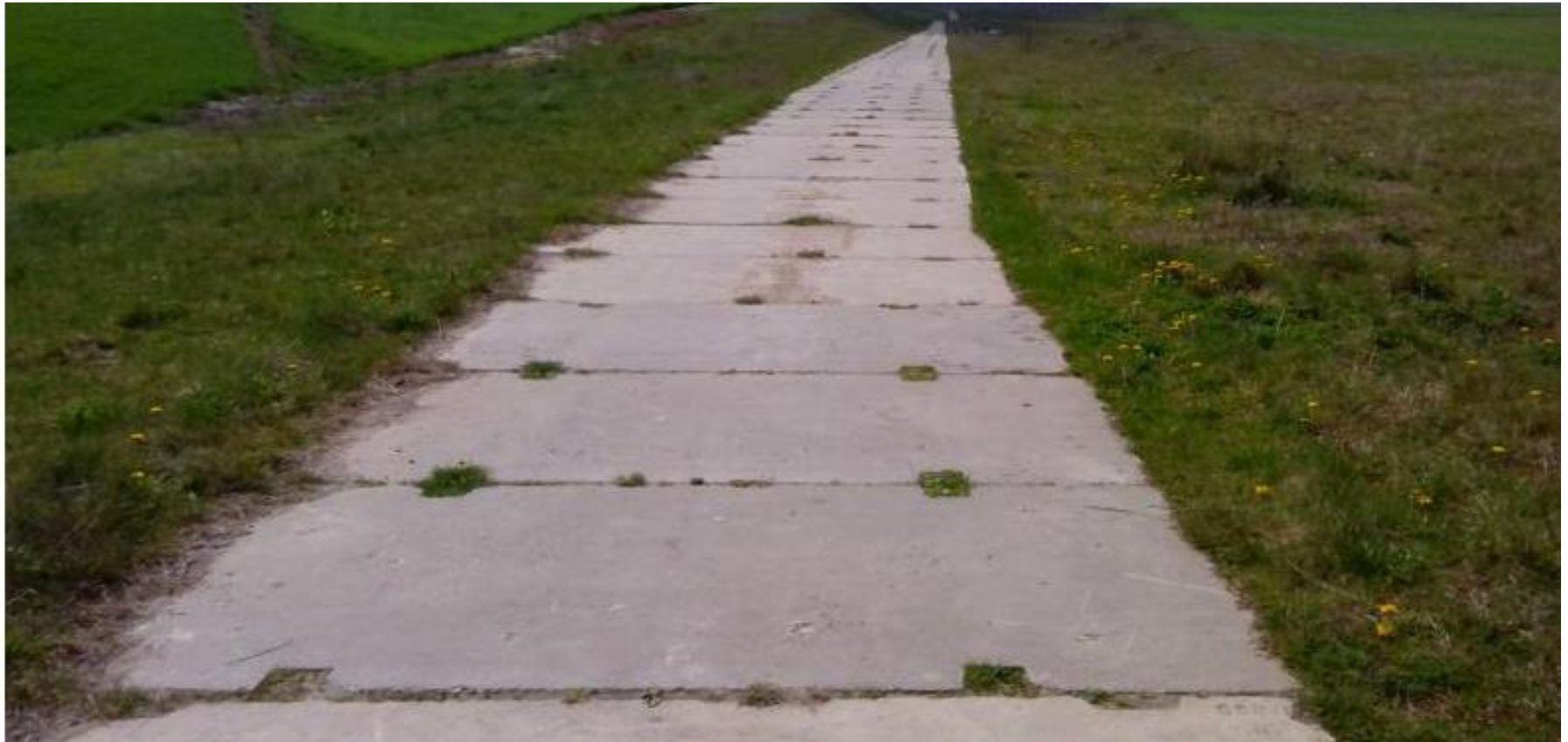
concrete slab road
