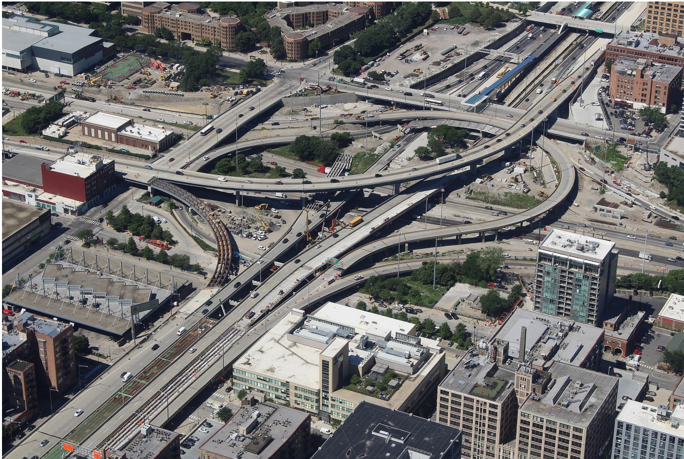
The Jane Byrne Interchange in Chicago, Illinois, a notable turbine interchange. 41.875577^{\circ}\text{N } 87.645042^{\circ}\text{W}
