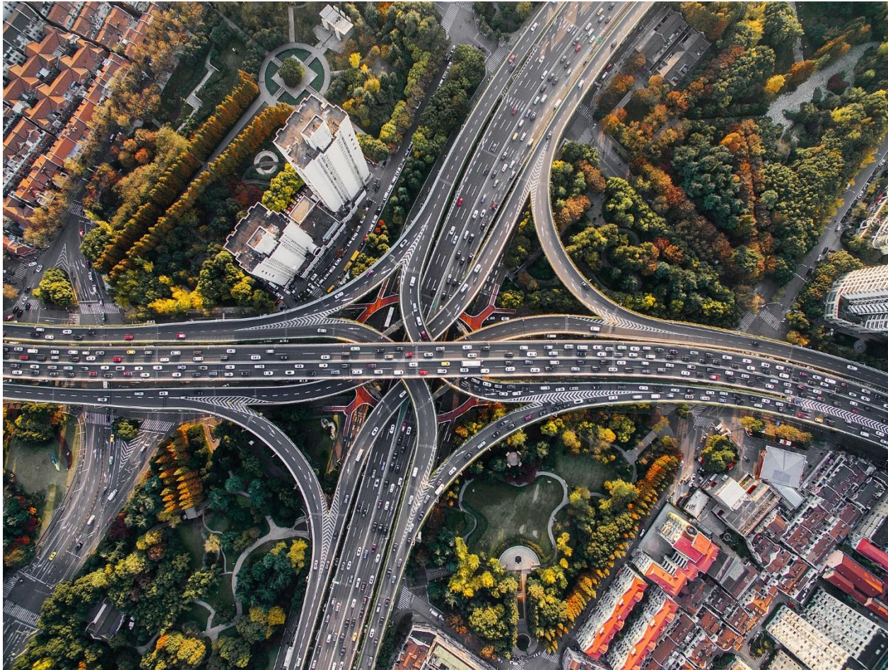
A multi-level stack interchange in Jing'an, Shanghai, China. 31.226335°N 121.464606°E
