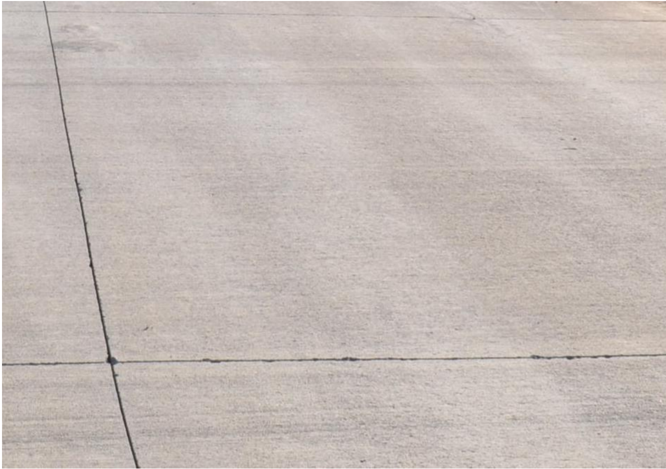
concrete road surface
