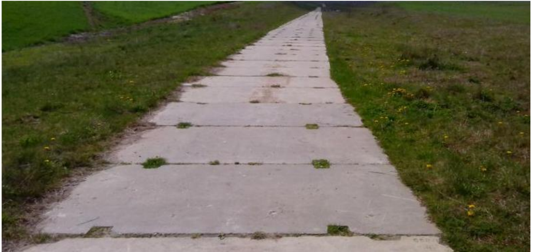
concrete slab road
