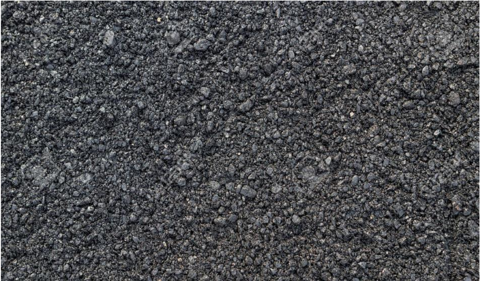
hot mix-asphalt road surface
