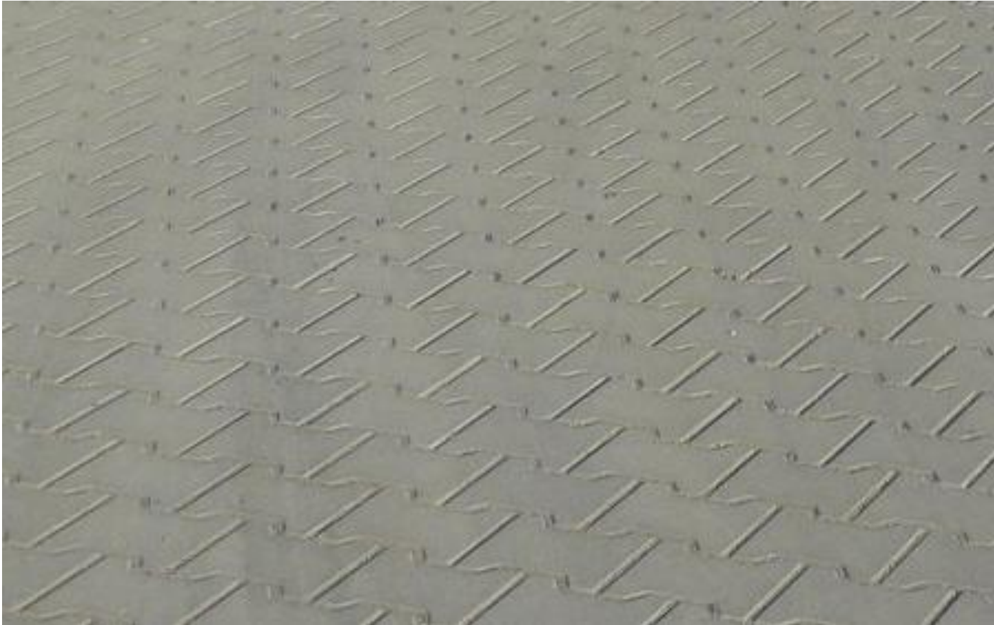
concrete setts road surface
