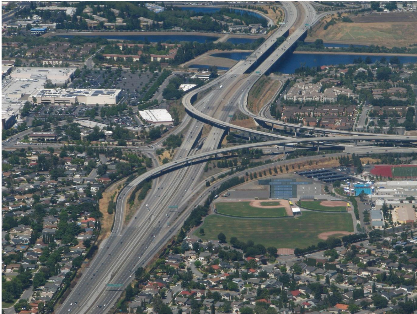
Complex T interchange of SR 85 and SR 87 in San Jose, California. 37.255721°N 121.858878°W
