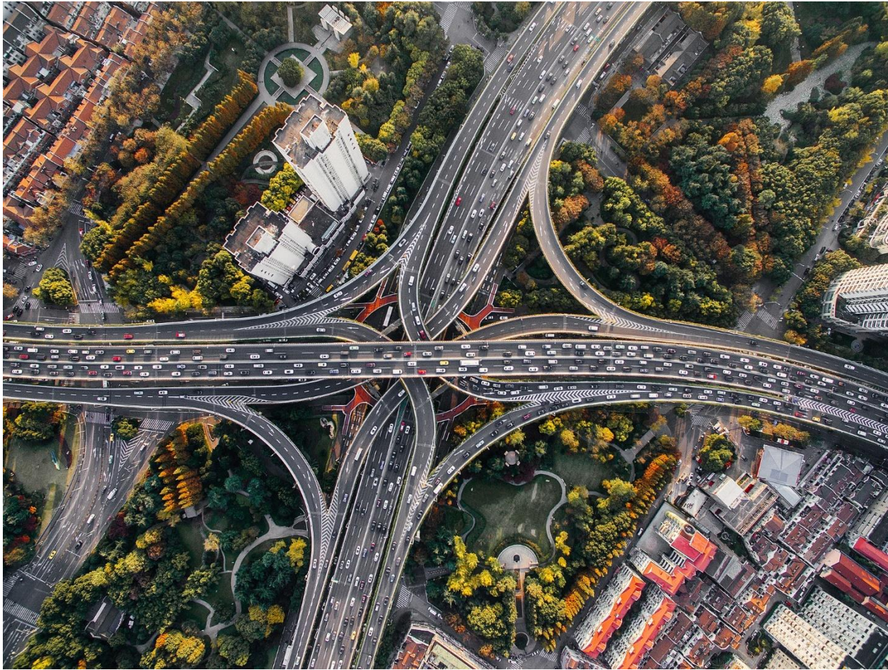
A multi-level stack interchange in Jing'an, Shanghai, China. 31.226335^{\circ}\text{N} 121.464606^{\circ}\text{E}
